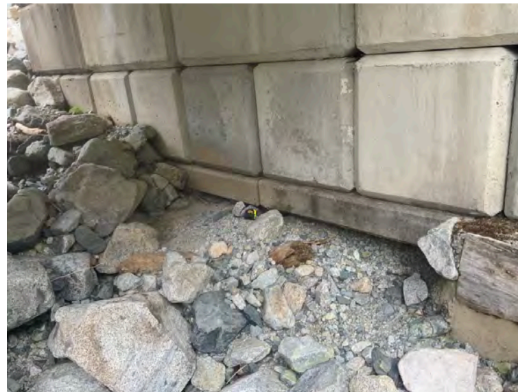
Left Bank Abutment when facing downstream
