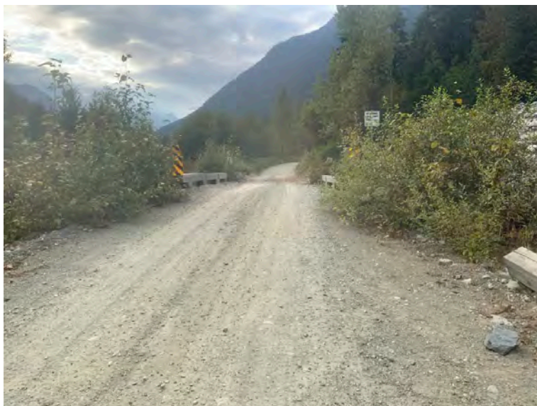
Approach from Left Bank when facing downstream
