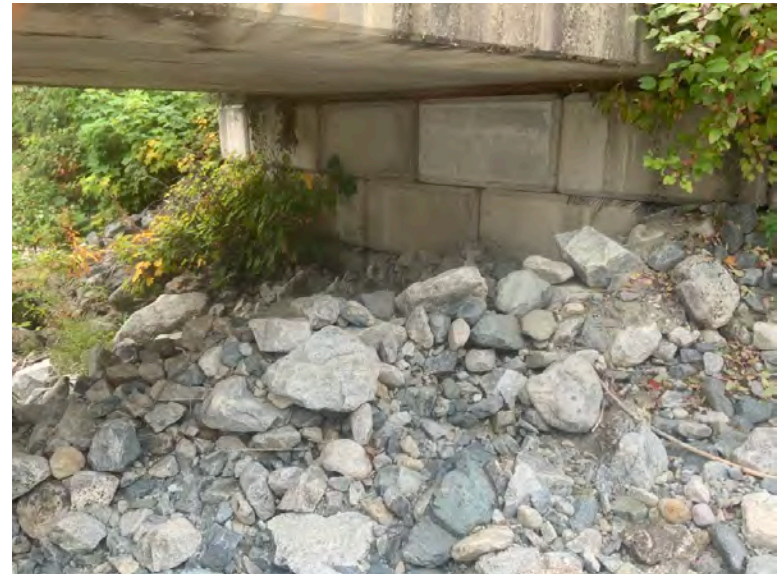
Right Bank Abutment when facing downstream
