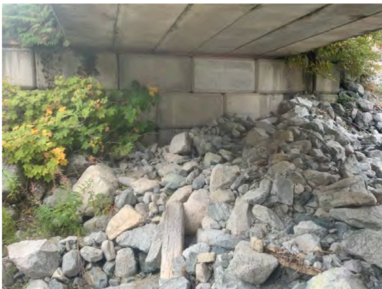
Right Bank Abutment when facing downstream
