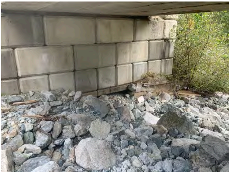
Left Bank Abutment when facing downstream
